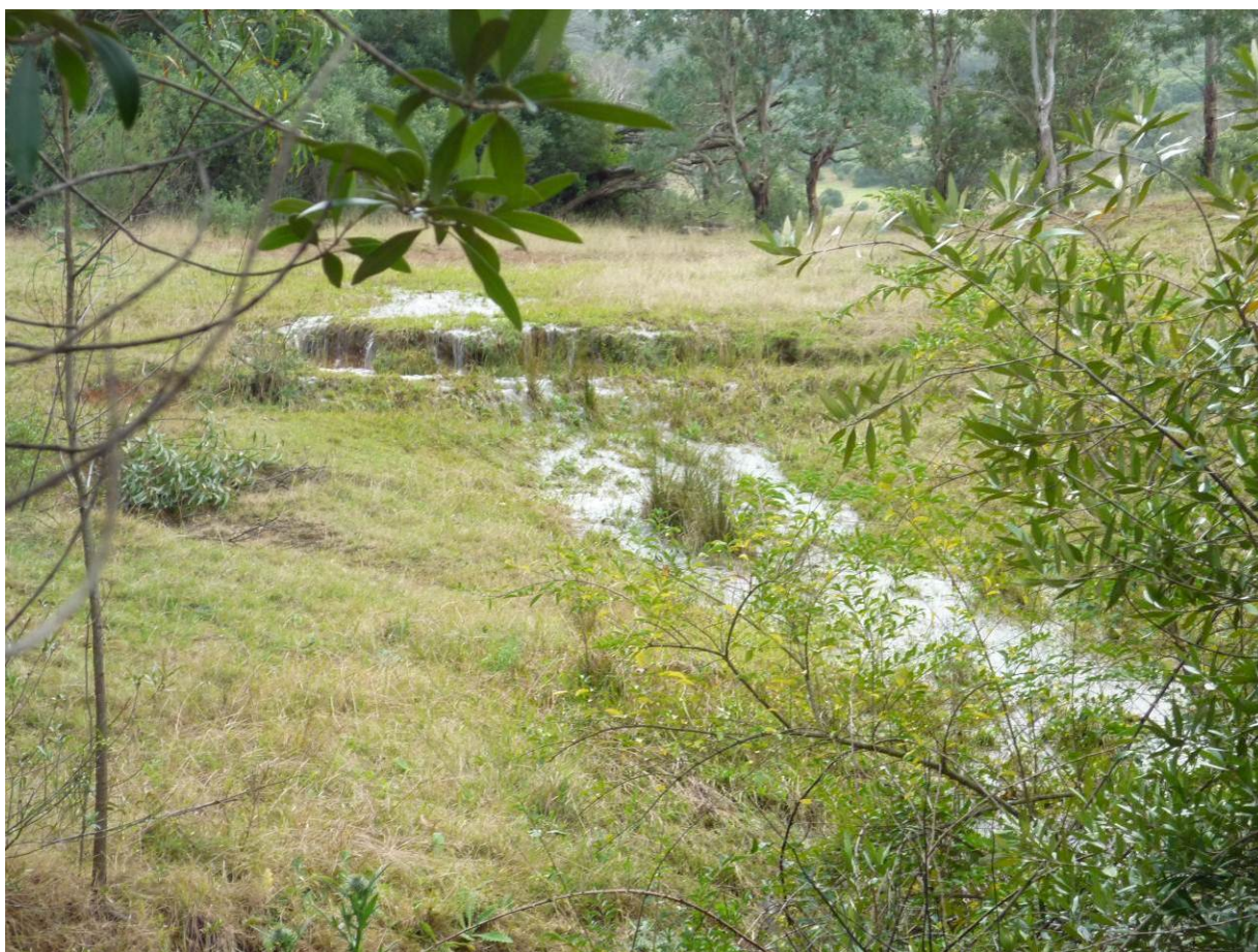
Photo 11 – Spillway for Dam 2 - requires stabilisation
