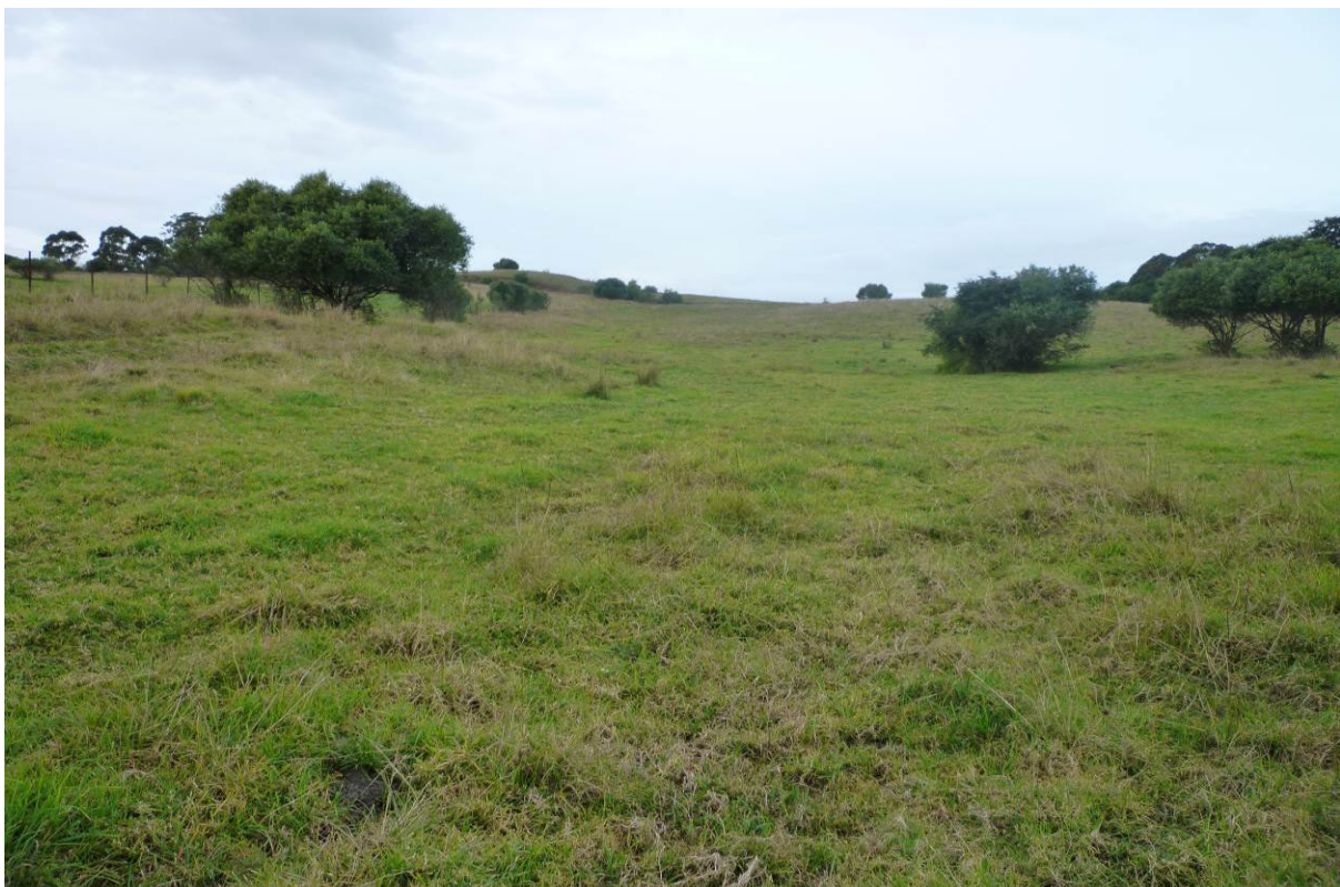
Photo 18 – Drainage line 4, grassed swale with no evidence of drainage < 12 hours after heavy rain
